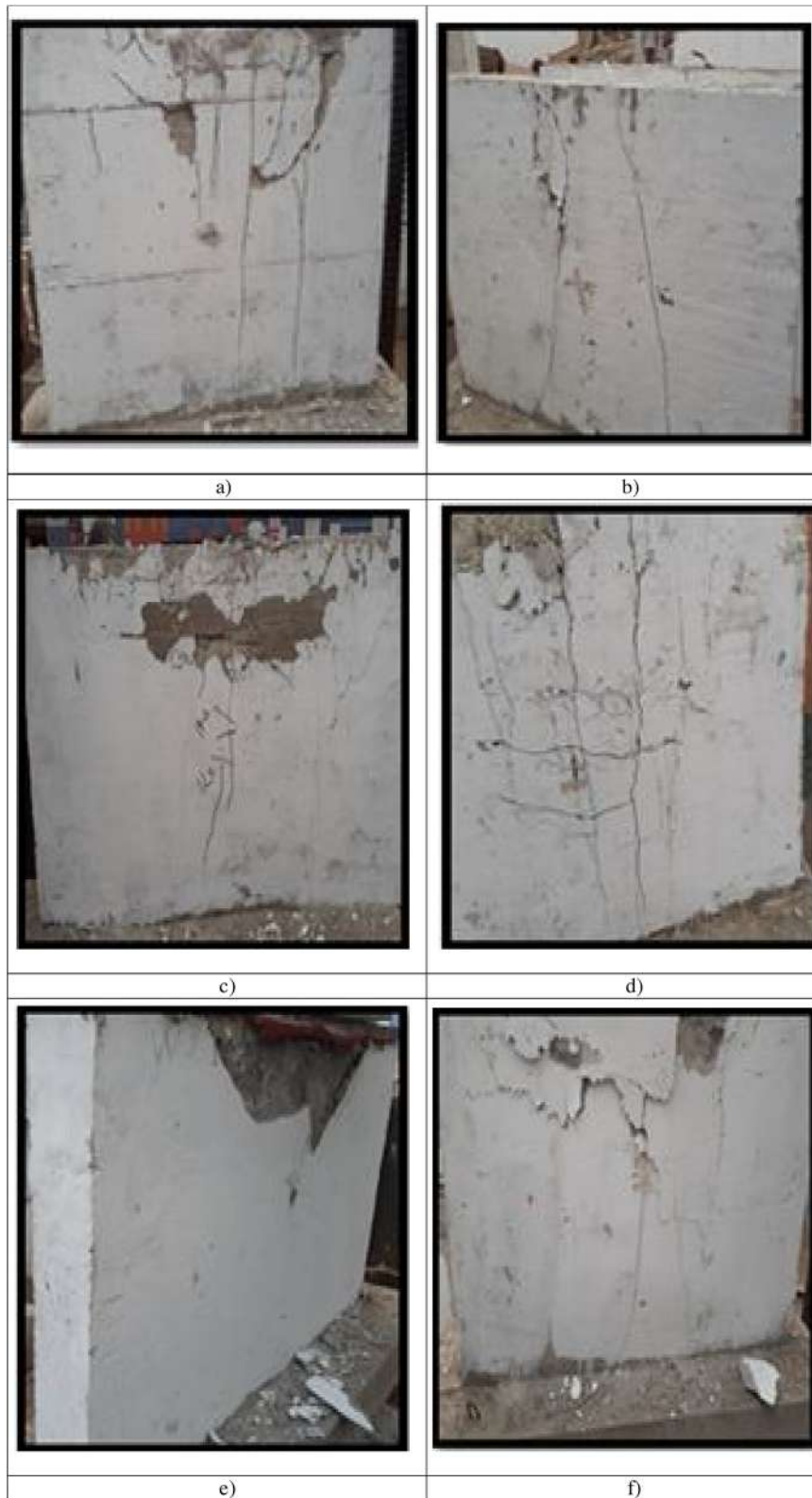
Fig. 9. Crack patterns of tested walls: (a) W1; (b) W1-2; (c) W1-4; (d) W2; (e) W2-2; (f) W2-4.
